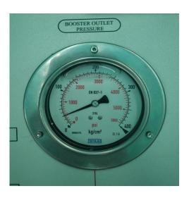
k. Boosting pressure at outlet is regulated by High pressure regulator (23).
